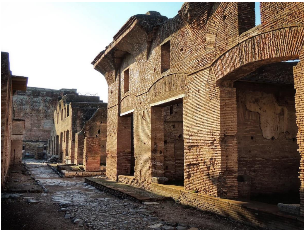
Large, multi-storeyed apartment building ( insula ), Ostia
